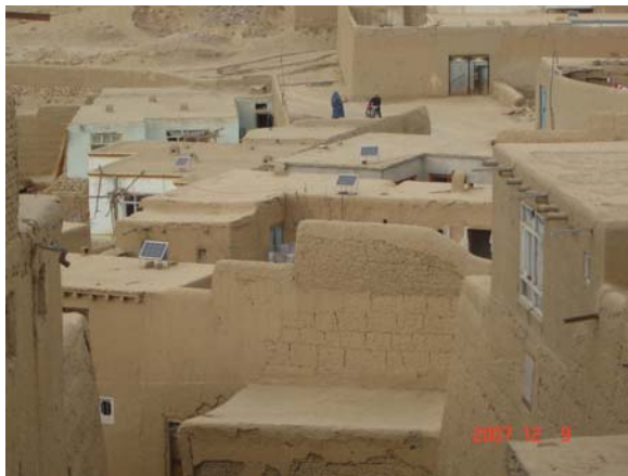
SOLAR HOME LIGHTING SYSTEM INSTALLED IN VILLAGE QALA-E-LUQMAN IN AFGHANISTAN
