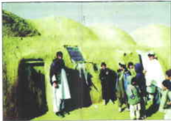
Solar Home Lighting System installed in remote village in Afghanistan
